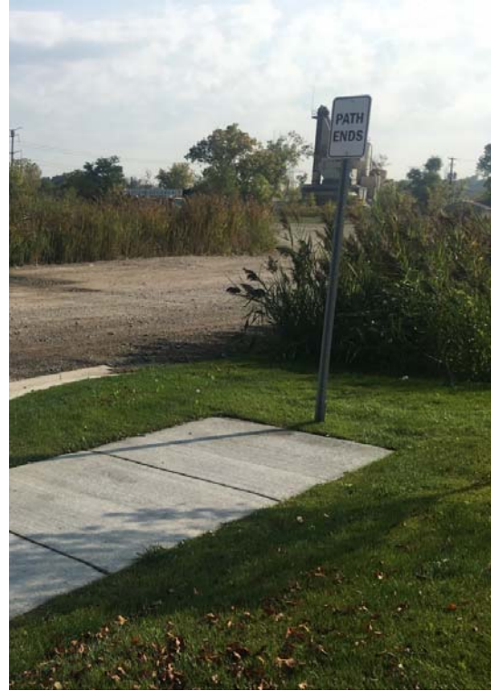
End of segment; possible extension in future
