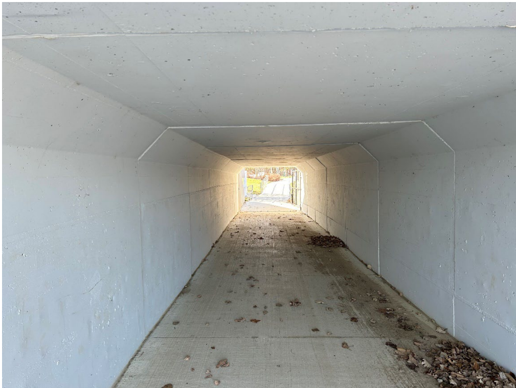
After – Inside tunnel
