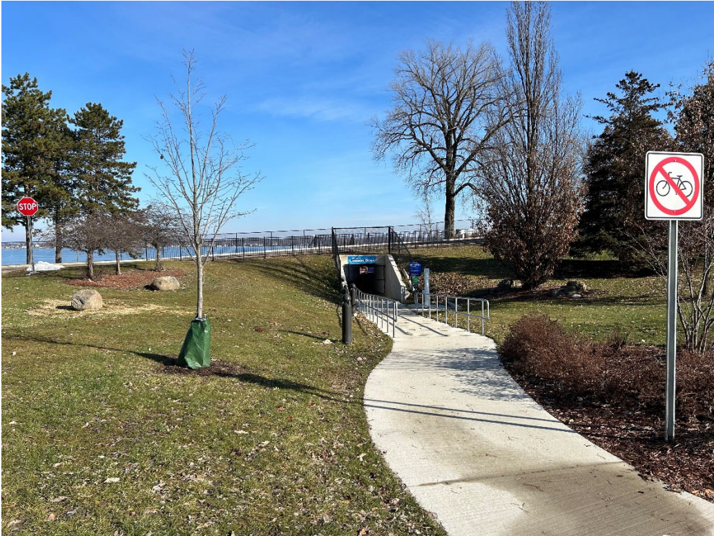
After – Park side (south)
