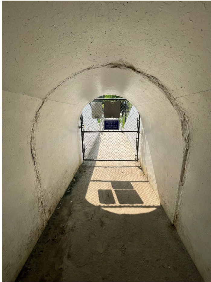
Before – Inside tunnel
