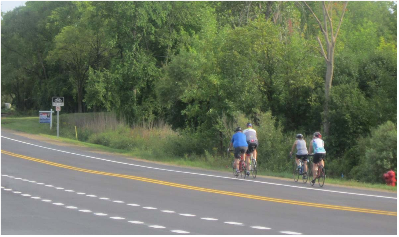
Taft Road Rehabilitation: Bike Lanes
