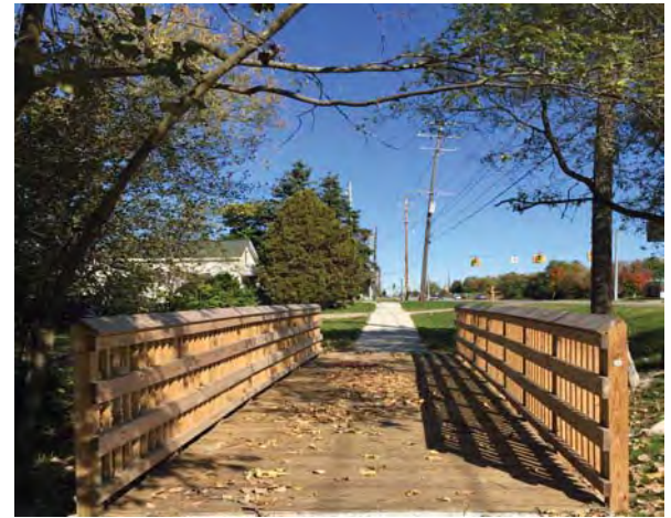
Pedestrian Bridge (On Novi Road between Nine Mile and Ten
